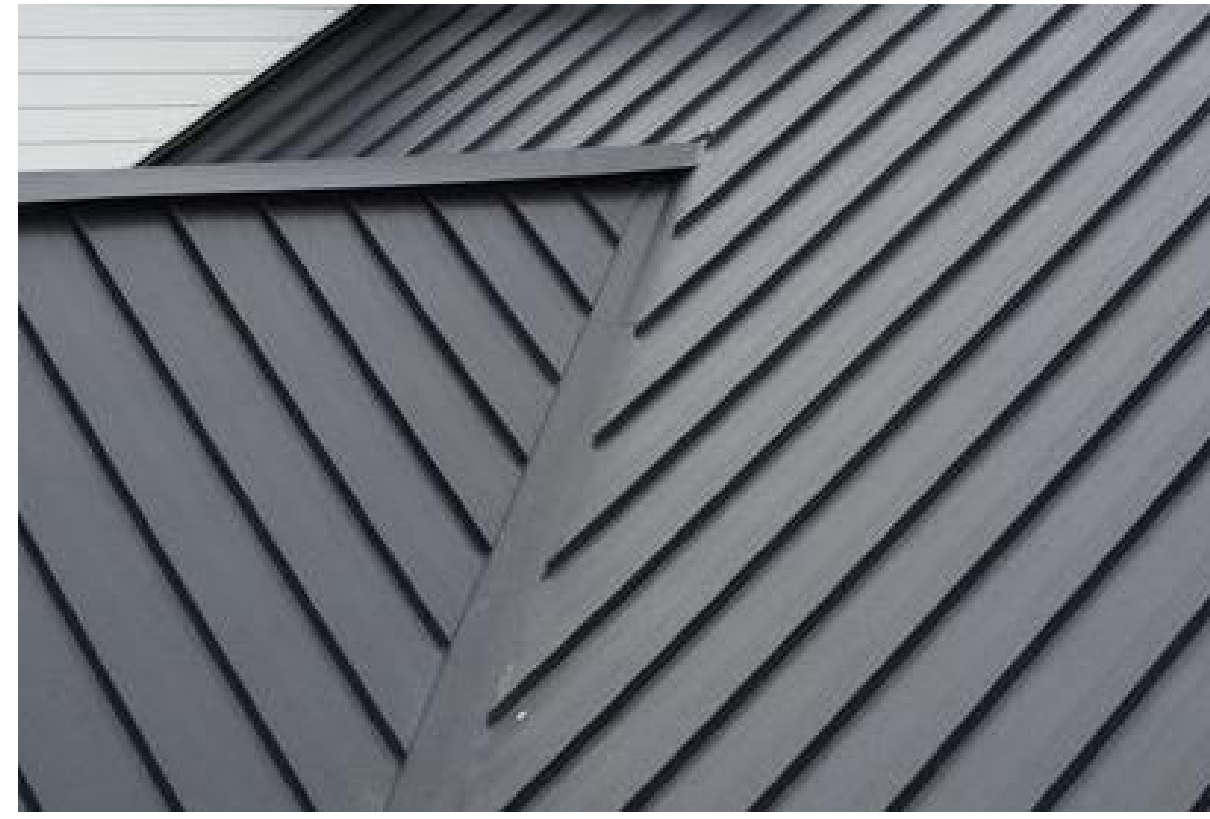
METAL STANDING SEAM ROOF
